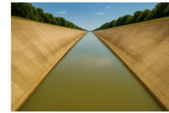
Large Drains & Canals
