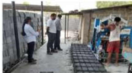
Ash to Bricks
