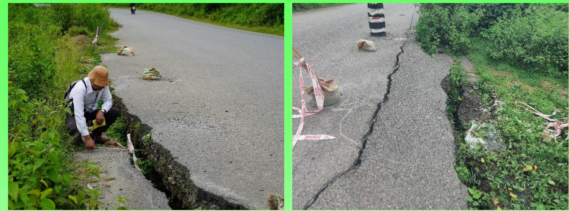
Fig. 21: Longitudinal open cracks (up to 25 cm wide) with vertical displacement (up to 30 cm) mapped along right edge of the pavement near Ch 115+867 km
