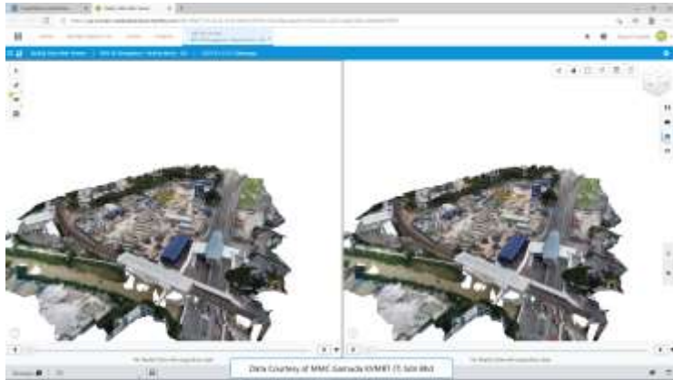
Compare construction progress using drones
