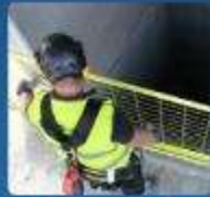
Open Shafts and Edges
