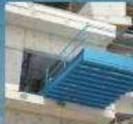
Unsafe Cantilever Loading Platform
