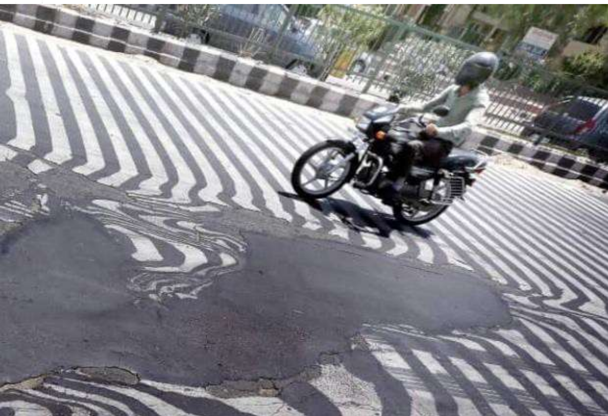
Melted asphalt of road in New Delhi during the heatwave in May 2015
